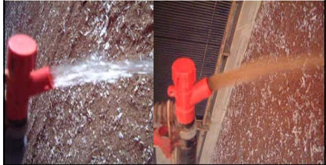
Line cleaned with acid
